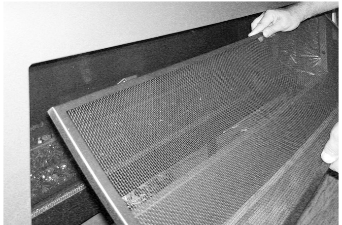
STEP 2: Angle the safety screen as shown on the picture and carefully bring into the fireplace opening.
