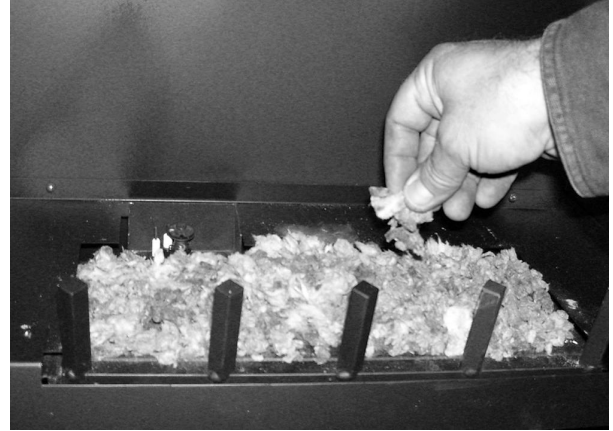
Figure 37 - Placement of Rock Wool on Burner
