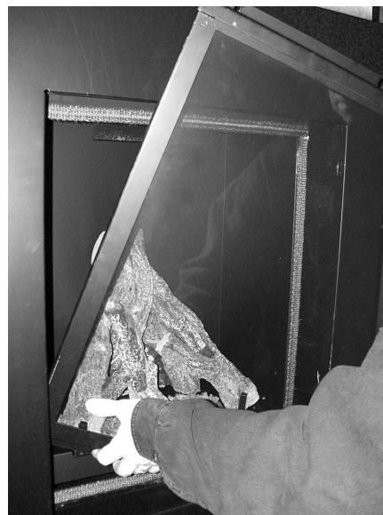
Figure 36 - Removing Glass Frame
