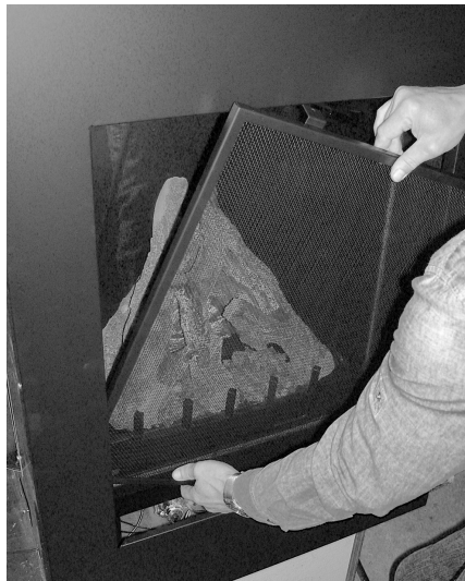
STEP 2: Angle the Safety Screen into the fireplace opening as shown above.
