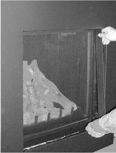
STEP 1: Insert the Right Side Panel into the opening angling in at the top.
