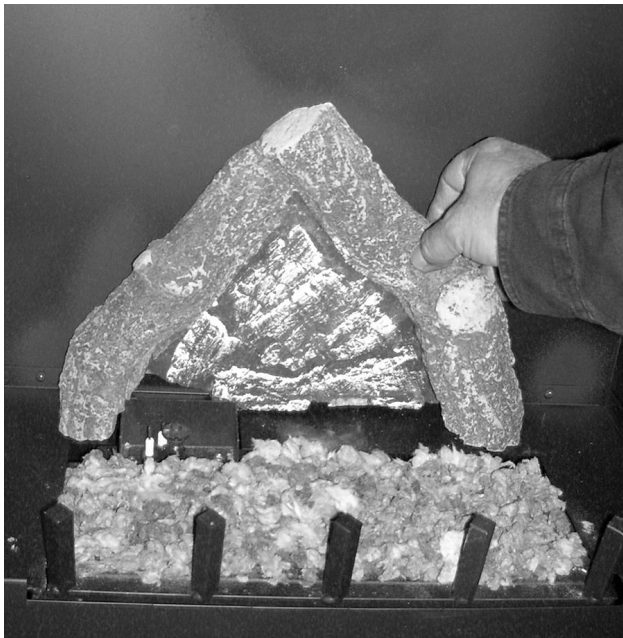
Figure 38 - Placing Rear Log (#1) on Log Support Bracket
