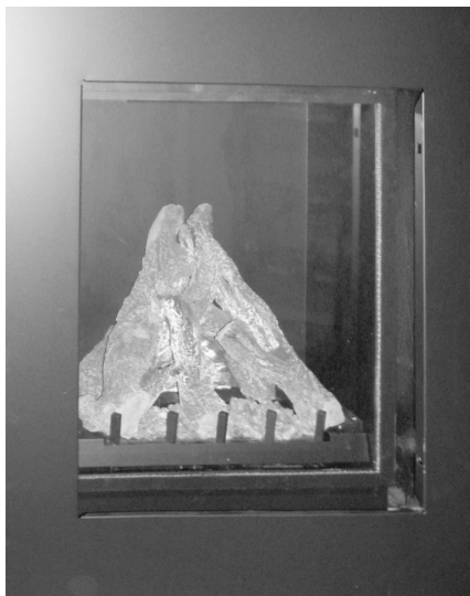
STEP 1: Remove Front Air Panel and both Side Panels from the fireplace. See next page for reference photographs.
