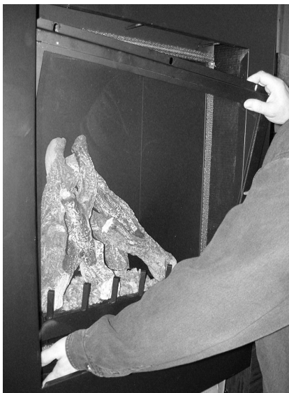
Figure 36 - Removing Glass Frame
