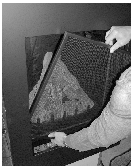
STEP 2: Angle the Safety Screen into the fireplace opening as shown above.
