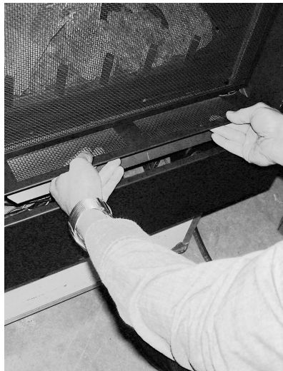
STEP 5: Support the Air Flow Panel on the left and right Side Panels.
