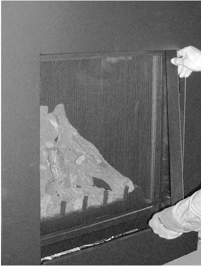
STEP 1: Insert the Right Side Panel into the opening angling in at the top.
