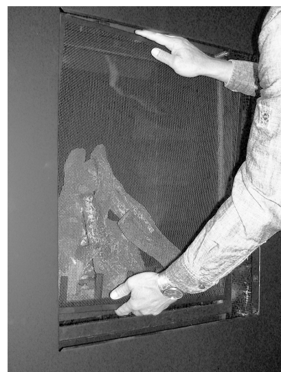
STEP 3: Lift the Safety Screen up so the tabs slide over the mounting bolts on the glass frame.
