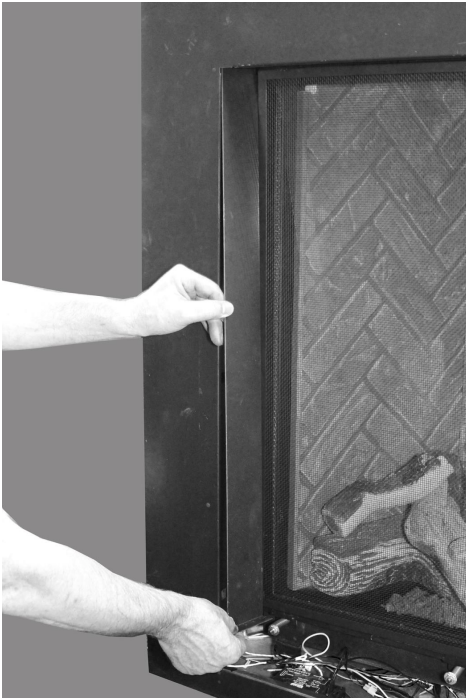
STEP 1: Insert the Right Side Panel into the opening angling in at the top.
