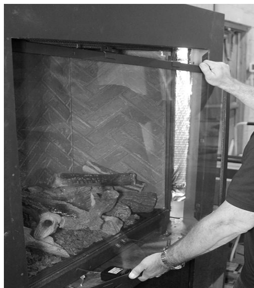
Figure 36 - Removing Glass Frame
