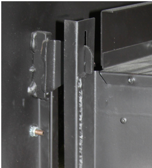
Figure 28 -Facing in place
