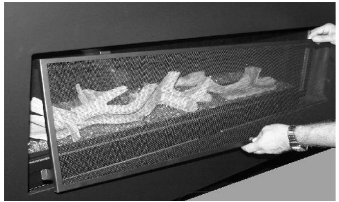
STEP 2: Angle the safety screen as shown on the picture and carefully bring into the fireplace opening.
