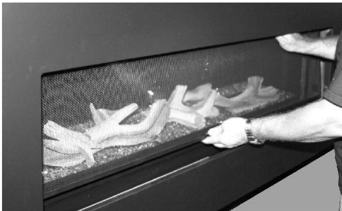
STEP 3: Position the safety screen inside of the fireplace in front of the glass door. Locate the two small vertical studs along the glass door frame bracket.
