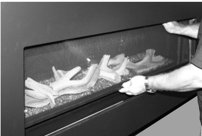
STEP 3: Position the safety screen inside of the fireplace in front of the glass door. Locate the two small vertical studs along the glass door frame bracket.
